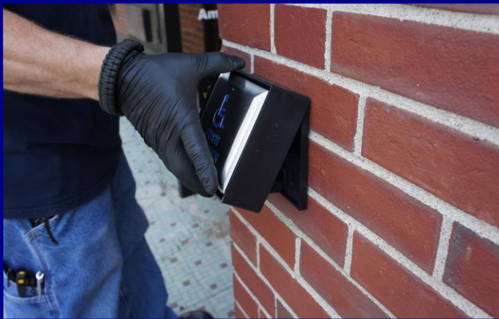
STEP 10: Re-install the cover.
