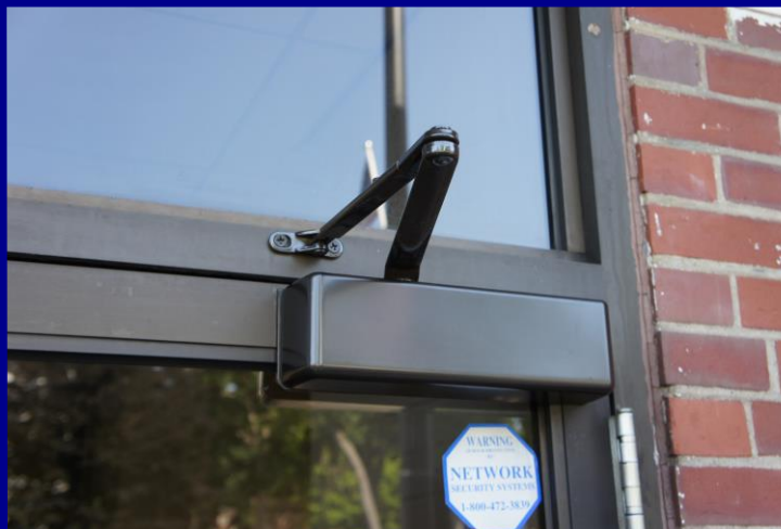
NOTES: A closer is required on the other side of the door to complete the open/close cycle due to the passive nature of our opener. Install the closer at this point.
