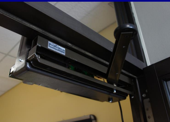
STEP 7-8: If necessary, perform field adjustments to sync the unit. The (2) field adjustments on the printed circuit board are "Time Hold Open" and "Load Sensitivity Adjustment".
